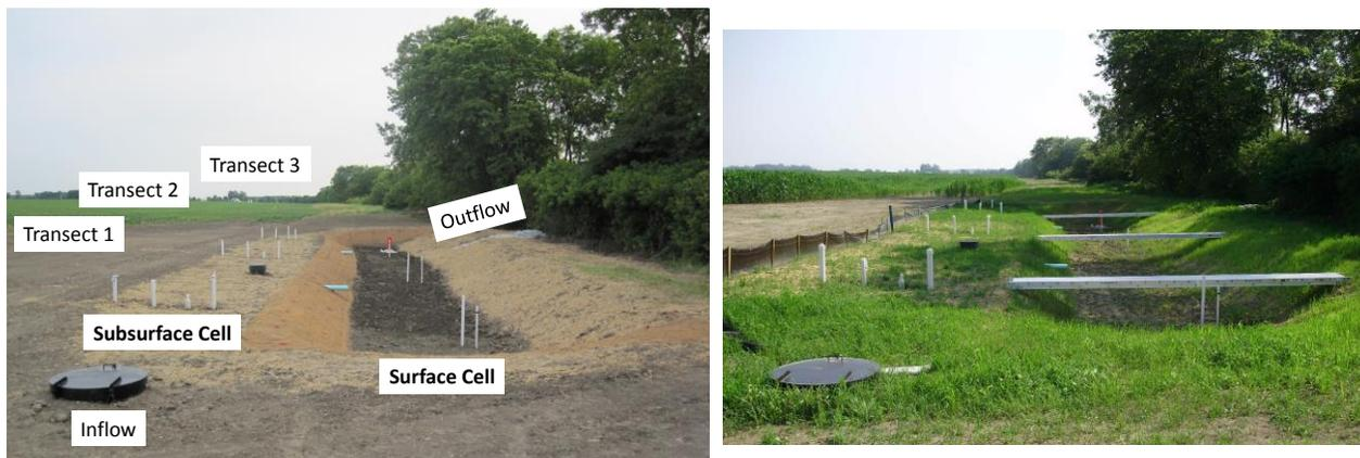
Fig. 4. The bioswale shortly after construction (*left*), and one month after installation (*right*).
