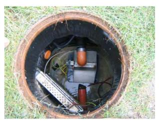
Constructed wetland outflow inspection chamber with water tip meter
