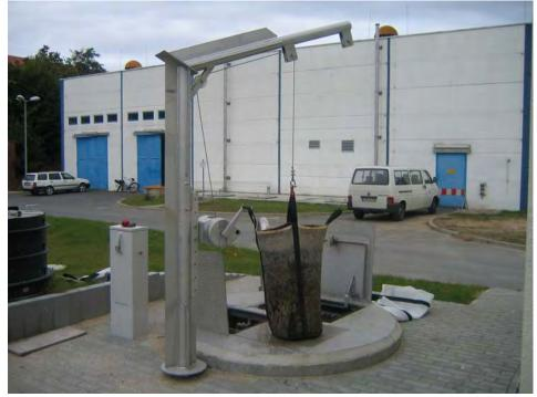
Fig. 2.4.11: Faeces dewatering facility including crane
